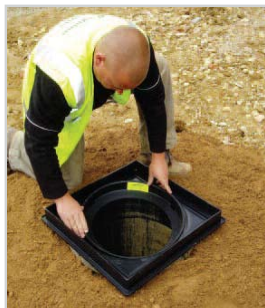
INSERTING THE CLKS 499 REDUCER
